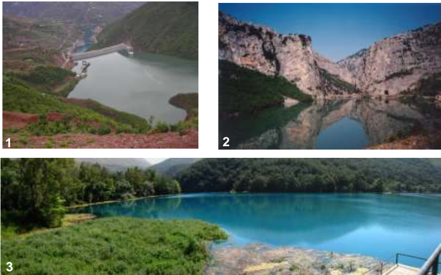
Figure 3-7: 1: Fierza dam and the reservoir at the Drini river in Bajram Curri; immediately downstream is the beginning of the Komani reservoir (June 2006); 2: the Shkopeti reservoir at Mati River in Miloti; 3: Bistrice Reservoir (Delvina) (Photos: A. Miho & L. Shuka).
