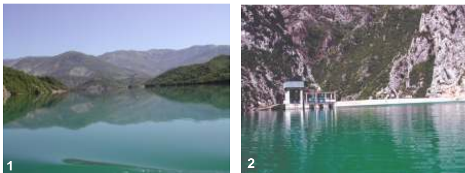
Figure 3-8: 1: Bovilla Reservoir (Tirana); 2: Dam of the Bovilla Reservoir with the water inlet to the Treatment Plant (Photos: A. Miho and L. Shuka).
